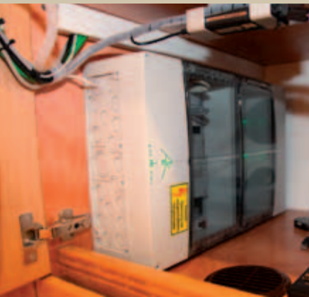
Ventilated, rubberized KNX® interface and line sub-distribution
